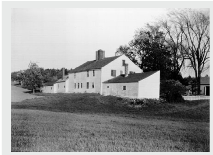
Old photograph shows rear of Houghton house and various additions.
