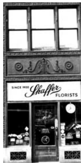
This finely detailed bronze storefront is typical of many constructed during the 1920s. The original grilles, spandrel panel
