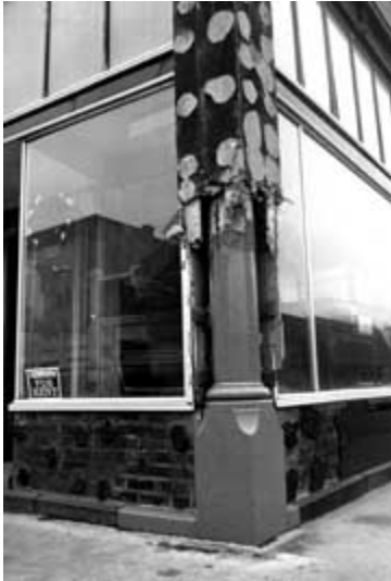
Storefronts of the 1940s, 50s, and 60s were frequently installed by attaching studs or a metal grid over an early front and applying new covering materials. Photo: Bob Dunn.
