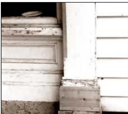
Rather than replace an entire wooden storefront, a new wooden component can be pieced-in, as seen in this column base. Photo: NPS files.
