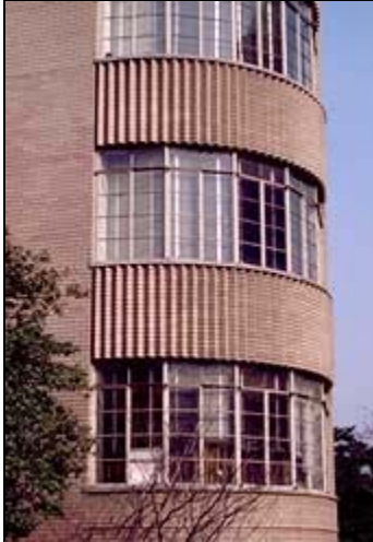
The historic steel sash is shown in place, prior to its removal and replacement with inappropriate aluminum sash (see below). Photo: NPS files.
