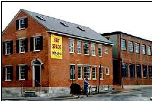
Two historic commercial buildings were successfully joined as part of a larger rehabilitation project. The glass connector detail is shown below. Photo: Martha L. Werenfels, AIA.
