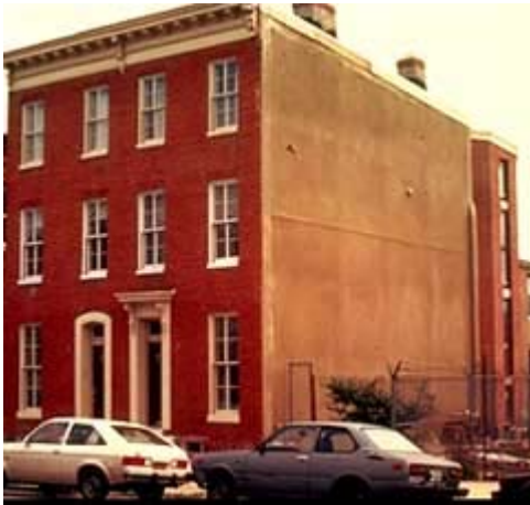
This new stair tower addition on the rear elevation of a historic townhouse is compatible in size, scale, and materials. This approach meets the Standards for Rehabilitation. Photo: NPS files.
