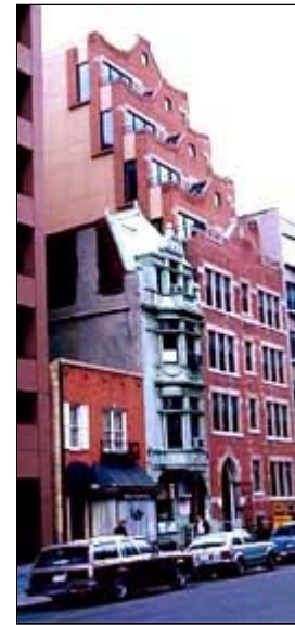
The historic character of this commercial building has been radically changed by a replicative four-story addition. This approach does not meet the Standards for Rehabilitation. Photo: NPS files.
