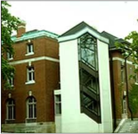
This new stairtower addition on a historic university building has been constructed on a highly visible side elevation. Together with its contrasting color and size, it obscures the historic form and roofline. This approach does not meet the Standards for Rehabilitation. Photo: Martha L. Werenfels, AIA.
