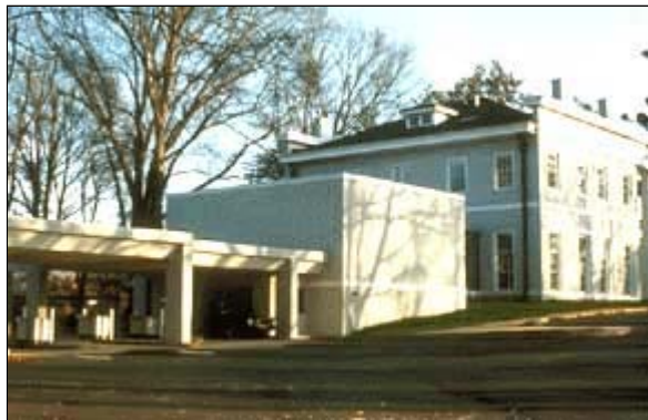
A sizeable addition was placed on a non-significant rear elevation of a late-19th century Greek Revival house that was rehabilitated for use as a bank with a drive-up component. The old building and new addition were sensitively joined by a small connecting hyphen. This approach meets the Standards for Rehabilitation. Photo: NPS files.
