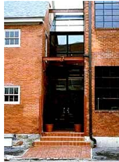
This small glass connector between two historic buildings is appropriately set back. This approach meets the Standards for Rehabilitation. Photo: Martha L. Werenfels, AIA.
