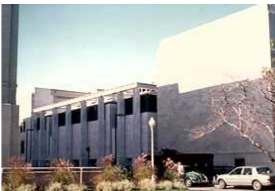
A contemporary new addition (above left) was designed to fit into a nonsignificant U-shaped area on a rear elevation of a historic library building. Note the new addition is lower than the historic building and clearly differentiated in
