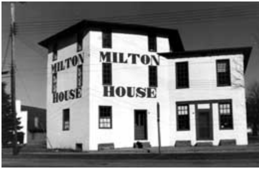
Milton House, Milton, Wisconsin (1844) is an early example of gravel wall construction with 12-to-15-inch thick monolithic concrete walls coated on the exterior with stucco. Photo: William Coney.
