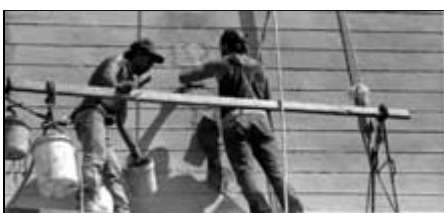
Workmen are applying patching concrete and using a trowel to form
