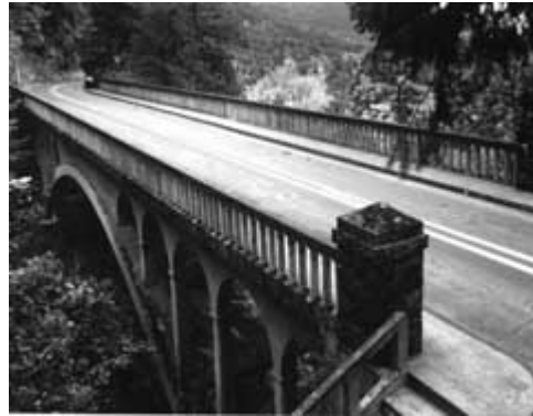
The new concrete spindles have been installed. This sensitive rehabilitation of the Young Creek Bridge (1914), part of Oregon's Columbia River Highway, re-used the historic concrete cap railing and stone piers because they were still in good condition. Photo: James Norman.
