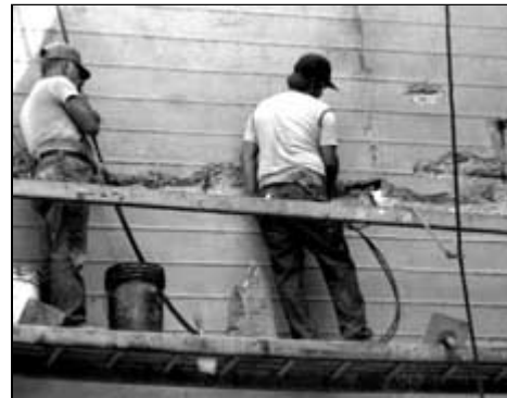
Deteriorated or redundant reinforcing bars are removed after evaluation by a structural engineer. An acetylene torch is being used to cut out the bars. Photo: NPS files.
