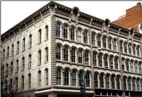
The historic cornice was successfully replaced with a fiberglass cornice. Photo: NPS files.
