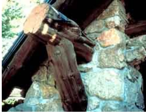
An inert material was injected into the hollow outrigger, permitting the outer wood to be retained and preserved.
