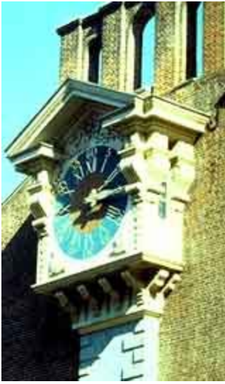
In the reconstruction of the clock tower at Independence Hall, the substitute materials used were cast stone and wood with fiberglass and polyester bronze ornamentation. Photo: NPS files.
