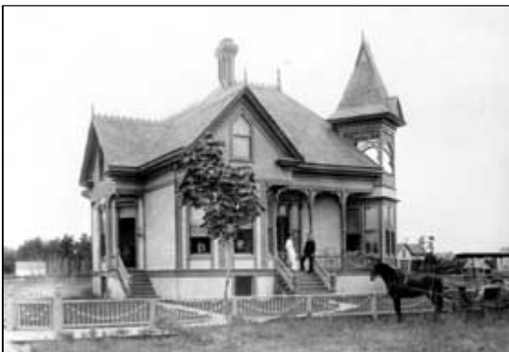
Readily available and inexpensive sawn shingles were used not only for roofs, but for gables and wall surfaces. Photo: Lane County Historical Society.
