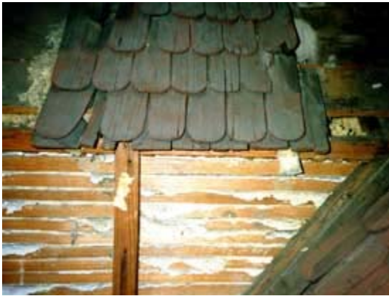
These weathered historic 19th-century handsplit and dressed shingles were found in place under a later altered roof. See also, below. Photo: John Ingle.
