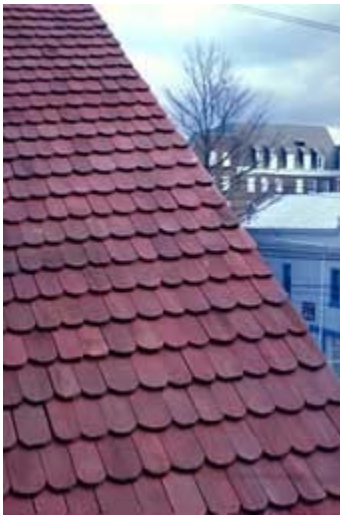
New rounded butt sawn shingles, with a smooth finish and red oxide stain, were used to replace the deteriorated shingles. The varying widths, between 4" and 7" will keep them from curling and cupping. Exposure length was determined from historic nail patterns on the historic spaced sheathing below. Photo: NPS files.
