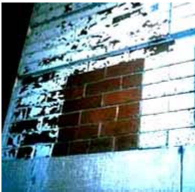
Any cleaning method should be tested before using it on historic masonry. Photo: NPS files.
