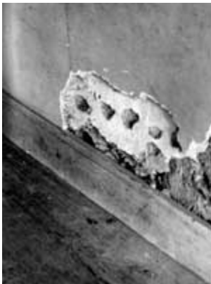
The builders of this mid-18th century house installed the baseboard molding first, then applied a mud and horse hair plaster. Lime was used for the finish plaster. Photo: NPS files.
