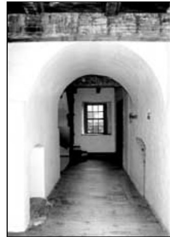
Schifferstadt, a simple house of German origin that dates to 1756, utilized plaster for both flat and curved walls. The building is located in Frederick, Maryland Photo: NPS files.
