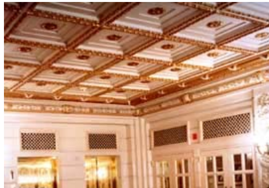
The elaborate coffered ceiling was designed for the Willard Hotel in Washington, D.C. (1902-04) by Henry Janeway Hardenbergh. It was restored as part of a rehabilitation project in the 1980s. Photo: Carol M. Highsmith.
