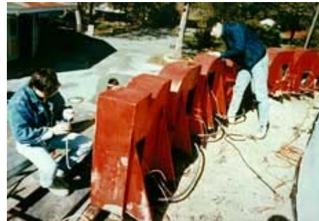
Workers prepare the "metal cans" from a sign for re-mounting. Photo: Larry Kanter.
