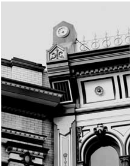
This shows a detail of a polychromed cast-iron facade in Petaluma, California, 1886 (O'Connell and Lewis, Architectural Iron Works, San
