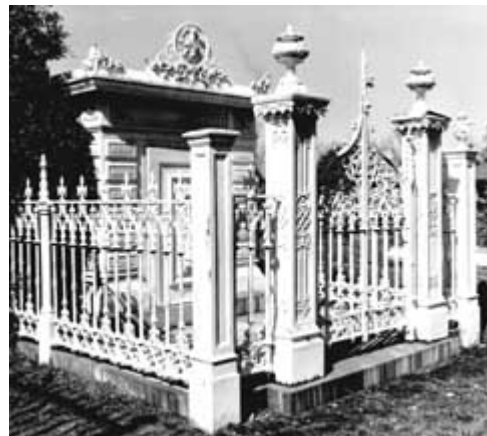
The Slatter Family Tomb in Mobile, Alabama, consisting of a cast-iron mausoleum and fence, exhibits the wide range of uses of the material in the 19th century. Photo: Jack E. Boucher, HABS Collection.
