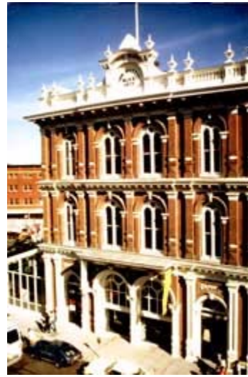
The west facade of the New Market Theater retains its original cast iron features.
