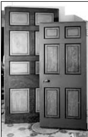
Historic doors may have graining patterns or clear finishes under one or several coats of plain paint, such as these restored 18th and 19th century doors. Photo: Jack E. Boucher, HABS, NPS.
