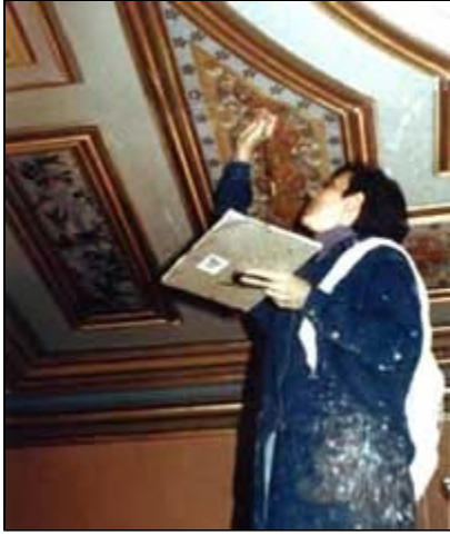
Traditional water-based paint and artists' brushes are being used to reproduce historic finishes within a restoration project. Photo: Courtesy, Alexis Elza.
