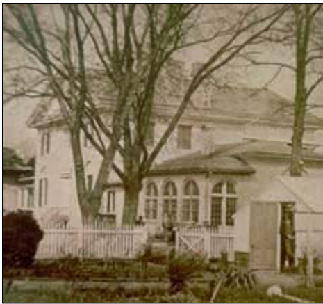
Prior to a replacing a roof, historical documentation is gathered (such as photo documentation) to determine the roof configuration. Photo: NPS files.
