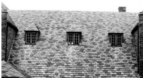
This graduated slate roof is composed of large, thick slates at the eave which are reduced in size and thickness as the slating progresses to the ridge. Photo: Jeffrey S. Levine.
