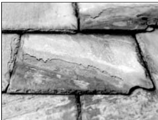
Paper thin lamination can be seen flaking off this weathered, 120 year piece of Pennsylvania Hard-Vein slate. Photo: Jeffrey S. Levine.
