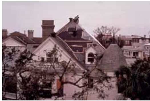
After a hurricane or other natural disaster, it may be necessary to stabilize a roof temporarily until materials can be obtained and a qualified roofing contractor hired. Significant slate roofs should not be stripped off and replaced with asphalt shingles. Photo: NPS files.
