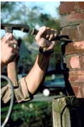
Here, a hammer and chisel are being
