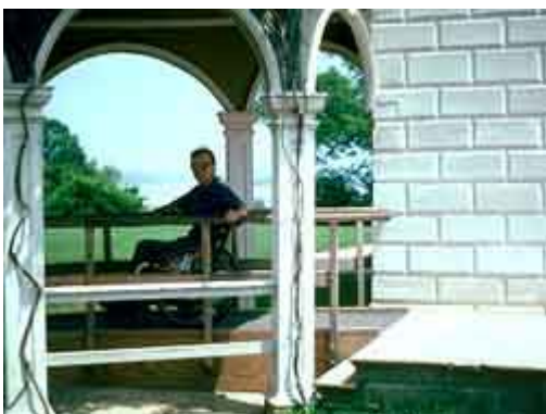
The significant building site is now accessible to people with disabilities (note steps in front of ramp). Photo: NPS files.
