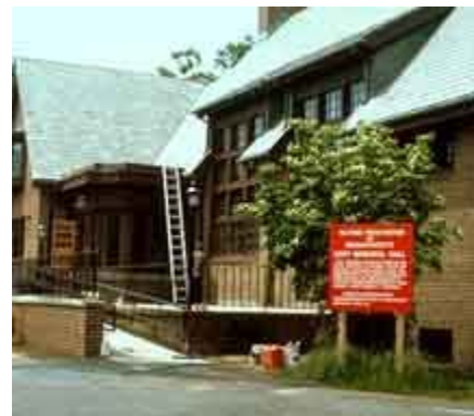
This accessibility ramp is compatible with the historic building in scale and materials. Photo: William Smith.
