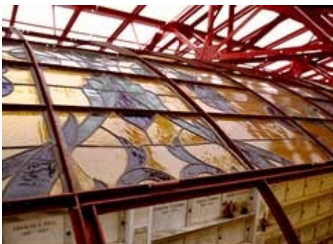
Before repairs began on the vaulted glass ceiling, a new diffusing skylight was installed to correct recurring leaks. Catacombs (ca. 1920), Cypress Lawn Memorial Park, Colma, California. Photo: Neal A. Vogel.
