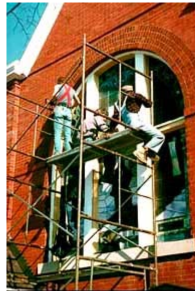
These workmen are performing exterior window maintenance after the protective glazing-- which had prevented maintenance--was removed. Photo: Neal A. Vogel.
