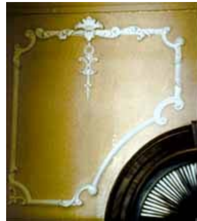
Based on documentary and physical evidence, missing composition ornament was re-created. Photo: Jonathan Thornton.
