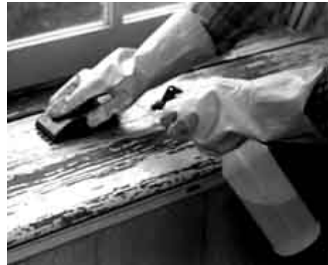
Wet sanding of interior surfaces will keep lead dust levels down, reduce the need for workers' protection, and provide a sound surface for repainting. Photo: NPS files.
