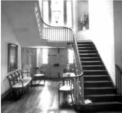
Significant architectural finishes should not be removed during a project incorporating lead hazard controls. Clear protective coatings may be added by conservators to areas subject to impact or abrasion. Photo: NPS files.
