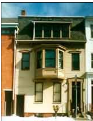
In this successful residential rehabilitation, deteriorated wood siding was removed from the foundation to the top of the first floor windows and replaced with matching wood siding. The building was repainted. Photo: Courtesy, Crispus Attucks Community Development Corporation.
