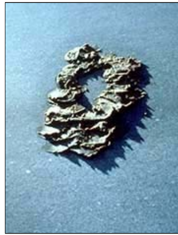
A poultice is often the preferred method of graffiti removal. Photo: NPS files.
