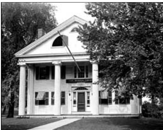
This 19th c. building in Massachusetts employed several energy-conserving features in its historic design, including shade trees, roof overhangs, awnings and shutters. Photo: HABS collection, NPS.
