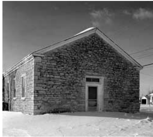
Heavy masonry walls and few windows serve to maximize warmth inside. Photo: HABS collection, NPS.
