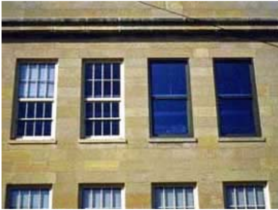
Tinted glazing has jeopardized the character of this historic office building and is, thus, not a recommended approach. Photo: Mike Jackson.
