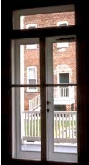
Storm doors have been added on the inside of this historic building as an energy-conserving device. Photo: NPS files.
