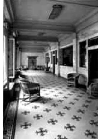
Ceramic mosaic tiles were practical for structures like this Bath House, Hot Springs, Arkansas (1914-1915). Photo: Jack E. Boucher, HABS Collection, NPS.
