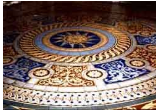
Encaustic floor tiles were decorated with traditional as well as original designs. Over time, the decorations can be worn thin by heavy traffic. Photo: NPS files.
