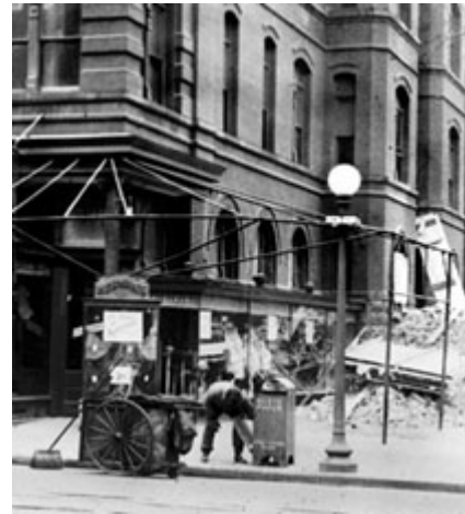
During the second half of the 19th century, iron plumbing pipe became a popular material for fixed awning frames. Here, a pipe frame without its canvas cover extends around the corner of a building in Washington, D.C. Photo: Library of Congress, Prints and Photographic Division, LC-USZ62-121160.
