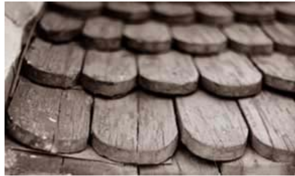
Replacement of particular historic details is important to the individual historic character of a roof, such as this rounded butt wood shingle roof. In the restoration, the drainage around a dormer was improved by the addition of carefully concealed modern metal flashing. Photo: NPS files.
