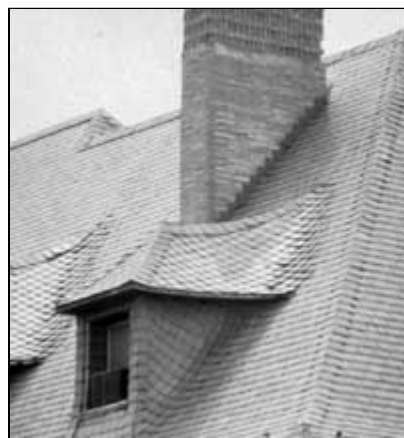
Because of the roof's visibility, the slate detailing around the dormers is important to the character of this structure. Photo: NPS files.
