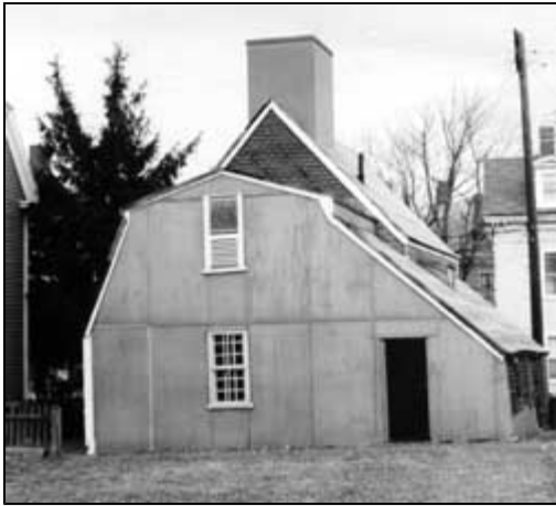
Temporary stabilization or "mothballing" with materials, such as plywood and building paper, can protect the roof of a project until it can be properly repaired or replaced. Photo: NPS files.
