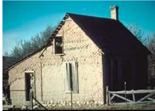
A traditional mixture of mud and straw plaster should be applied to stabilize the exterior of this house. Photo: NPS files.
