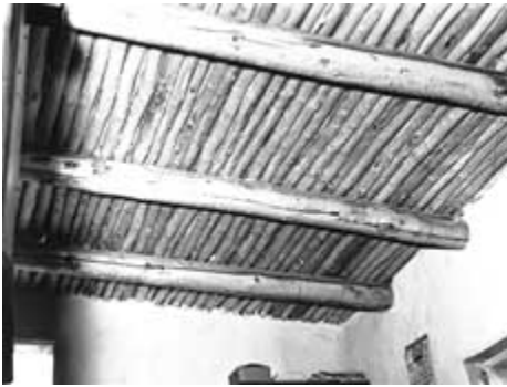
Viga logs and savinos are seen in the interior of the adobe building. Often the wooden materials that comprise the traditional flat adobe roof create interesting and pleasing patterns on the ceilings of interior rooms. Photo: Russell Lee, Farm Security Administration Collection, Library of Congress.
