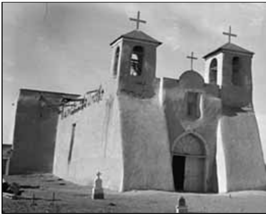
San Francisco de Assisi Mission Church in Rancho de Taos, NM, was constructed of adobe between 1772 and 1819 and, because of its distinctive sculptural quality, is one of the most famous and frequently photographed of the mission churches. Photo: HABS Collection, NPS.
