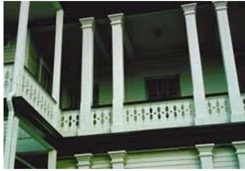
Decorative wood exterior or interior features should not be cleaned abrasively. Photo: NPS files.
