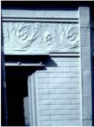
Decorative pressed metal interior or exterior features should not be cleaned abrasively. Photo: NPS files.
