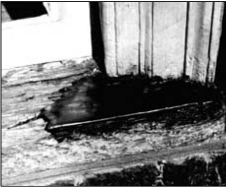
This illustrates a two-part epoxy patching compound used to fill the surface of a weathered sill and rebuild the missing edge. When the epoxy cures, it can be sanded smooth and painted to achieve a durable and waterproof repair. Photo: NPS files.
